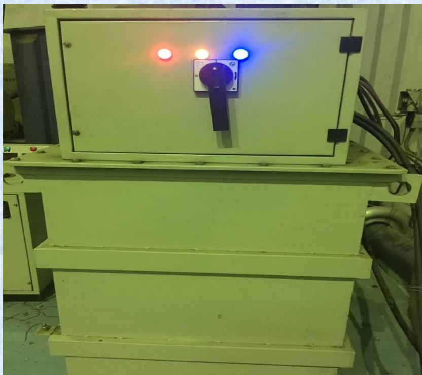
3-Phase Booster Transformer, 75 kVA, 2000 V & 52 Amps
